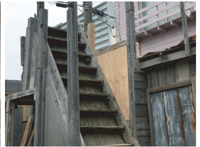
Savage Construction (still images), 2013-2024
